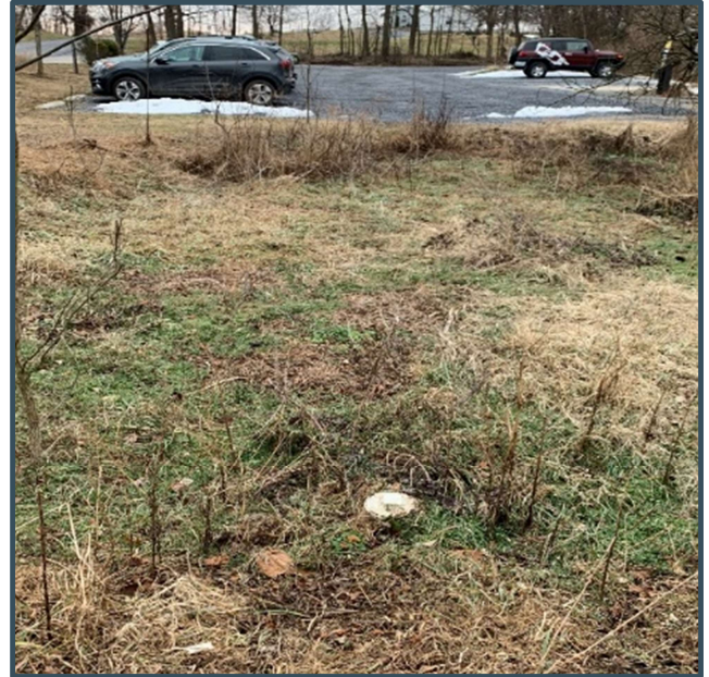
Figure 6: Site of parking lot expansion
