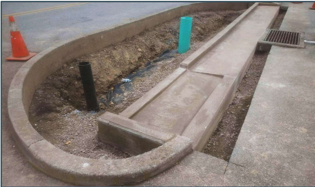
Figure 11: Example of sediment trap
