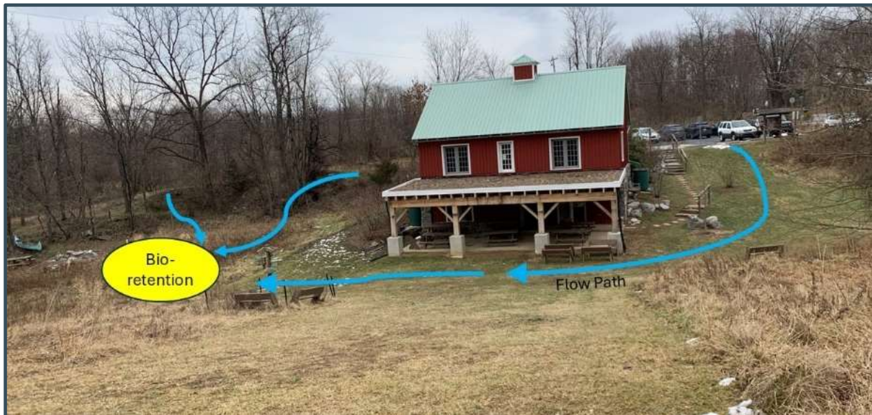
Figure 7: Flow path of Cool Spring surface water flow path
