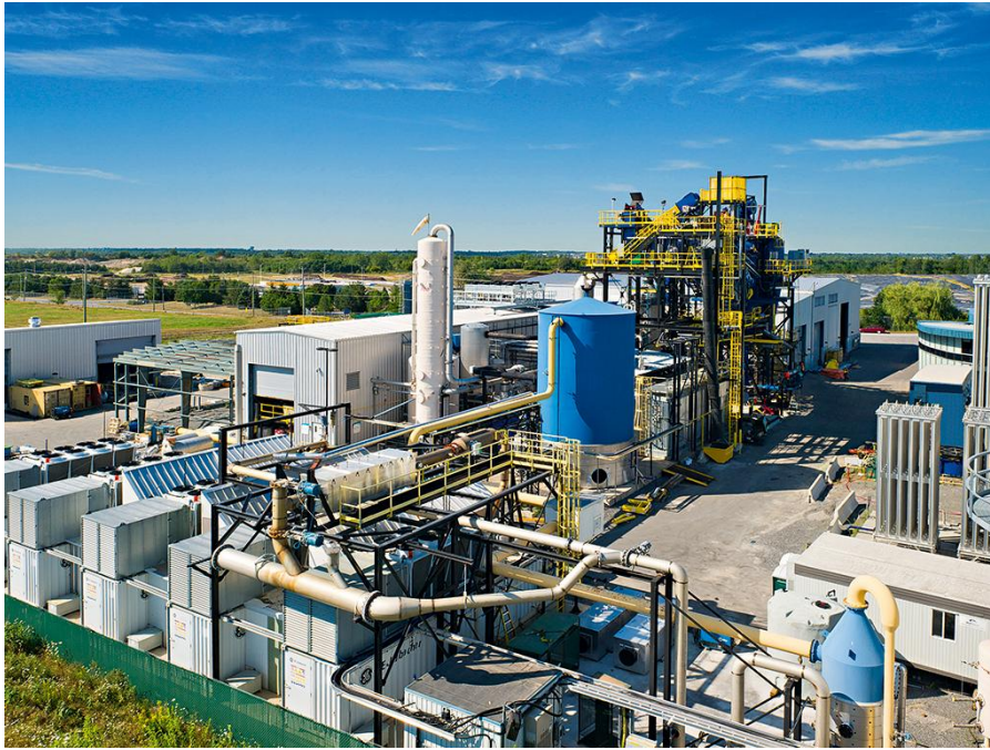
Figure 4: The Plasco facility
