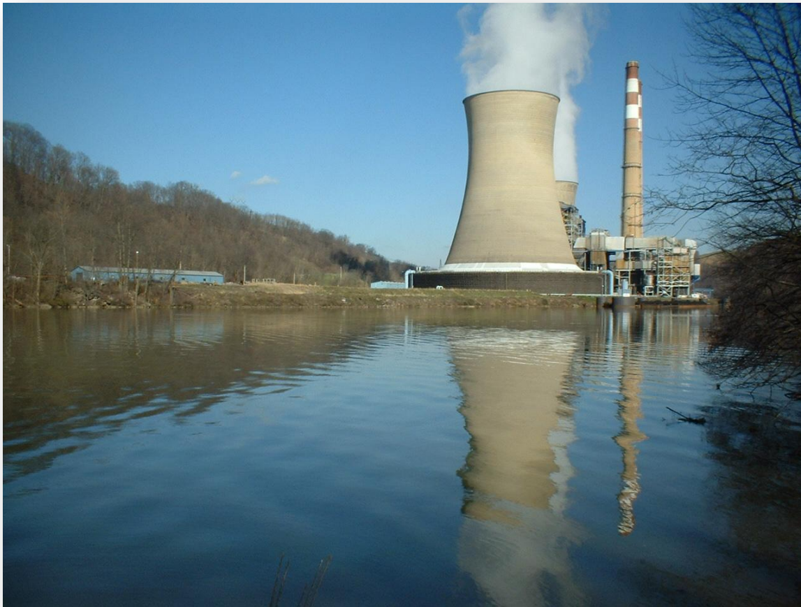
Figure ES-9: Fort Martin coal-fired power plant, West Virginia
