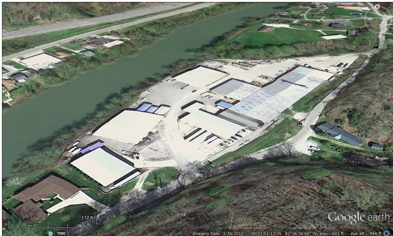
Figure 9: Possible potential significant contaminant source just downstream from the Freedom Industries site
