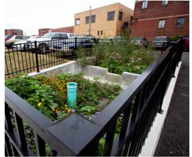
An example of green infrastructure, a rain garden in Beckley slows the flow of water into creeks and, eventually, the New River. The plants in the rain garden help filter pollutants from the water before it reaches the river.
