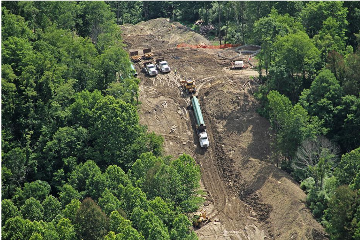
Figure 4: Steep slope construction of the Stonewall Gathering-Momentum pipeline in West Virginia
