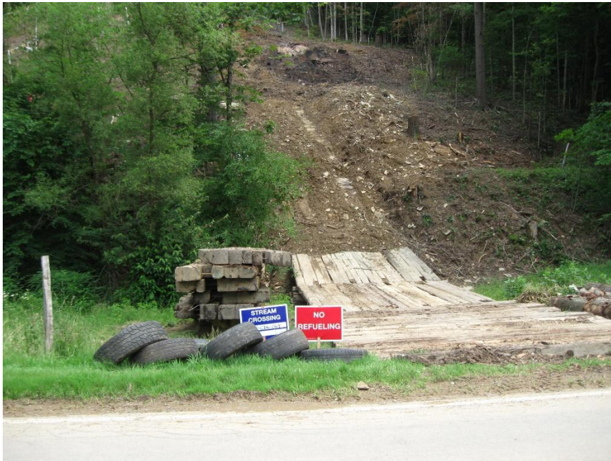
Figure 6: Constructing a pipeline stream crossing between Ireland and Flatwoods, West Virginia
