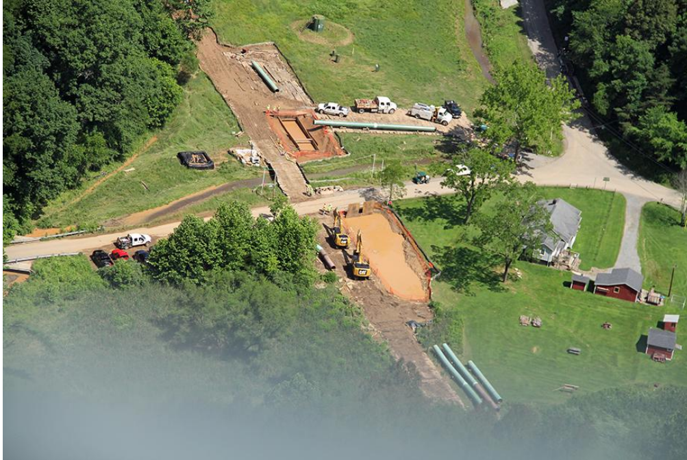
Figure 2: Construction of the Stonewall Gathering-Momentum pipeline in West Virginia
