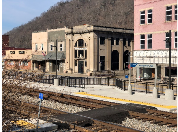
Montgomery Amtrak station (Downstream Strategies)
