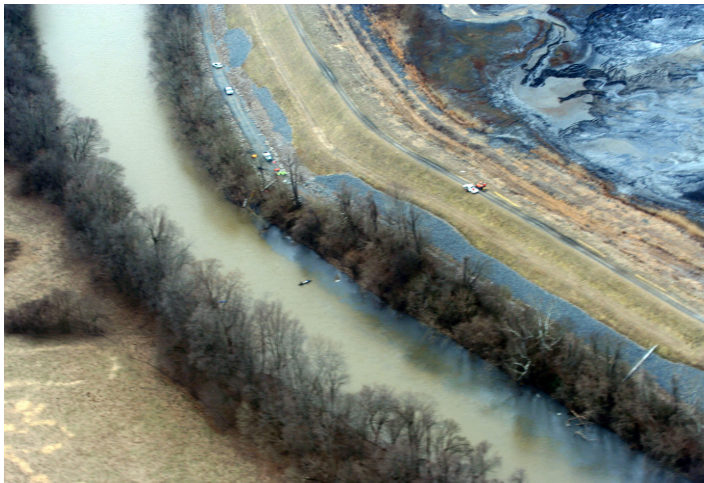
The rupture of a stormwater pipe at a former coal-fired power plant owned by Duke Energy spilled 27 million gallons of contaminated water and 39,000 tons of coal ash into the Dan River in February 2014. The disaster exposed the utility's negligence and drove policymakers to ensure all coal ash ponds in the state close safely by 2029.
