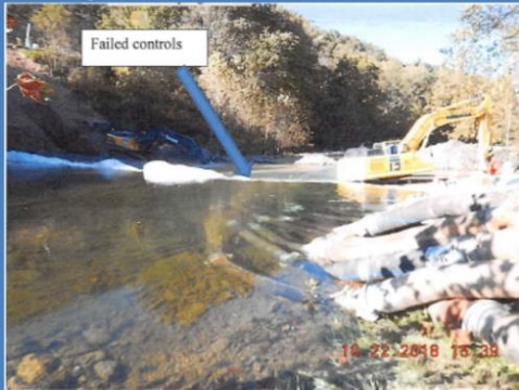
Failed dam with approximately 20 intake lines upstream of the dam
