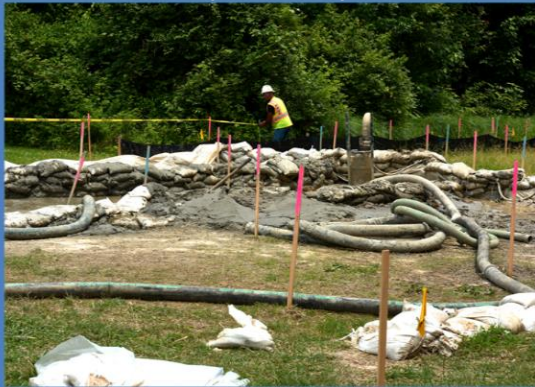
Drilling mud released during an IR in Middletown (Dauphin County)
