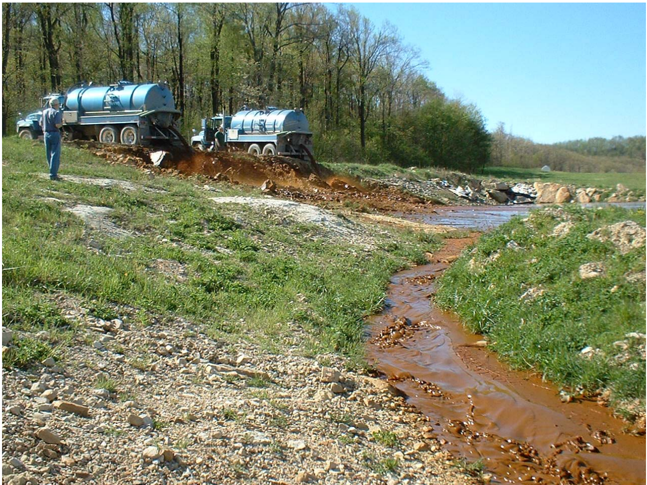
Figure 1: Tanker trucks unloading Omega mine sludge into F&M pits
