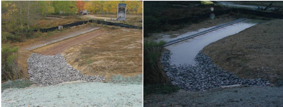
Figure 20: Level spreaders during construction and storm events
