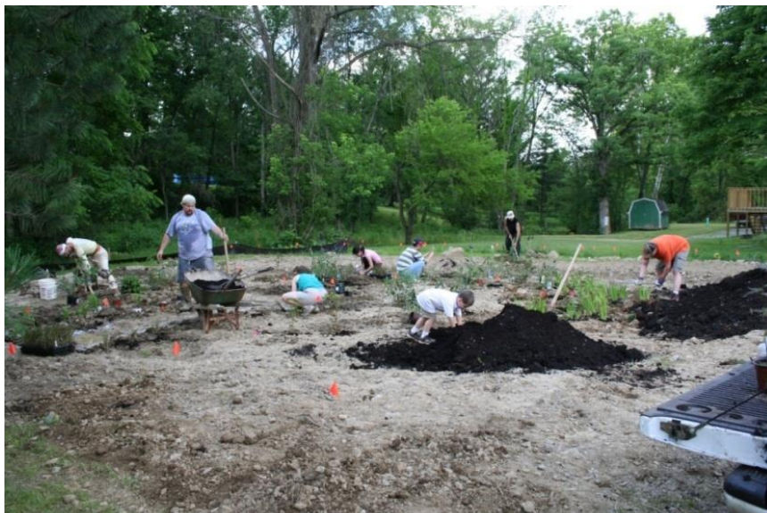
Figure 14: Building a rain garden in the Suncrest neighborhood
