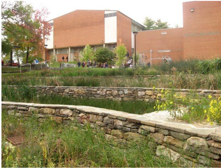
Figure 7: Terraced rain gardens at the Sidwell Friends School, Washington DC
