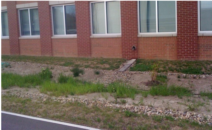
Figure 16: Bioswale along United States Department of Agriculture building in Morgantown
