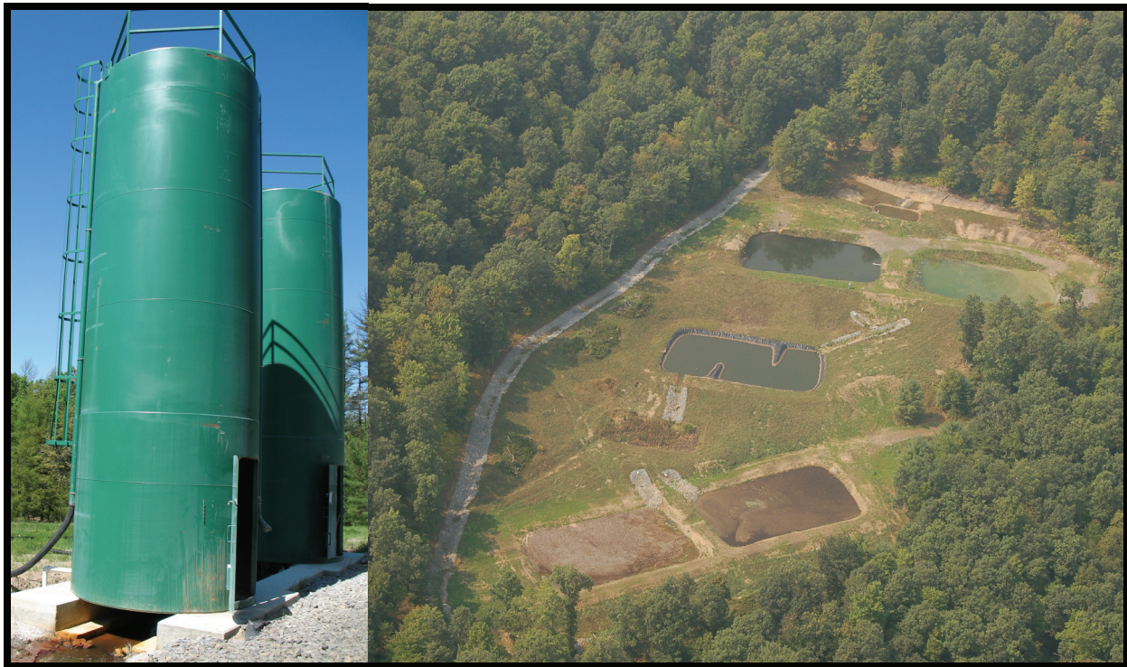
Note: Active system on left shows lime dosers on Porcupine Run in the Bennett Branch watershed. Passive system on right is on Middle Branch in the Kettle Creek watershed. Photo credits: Amy Wolfe.
